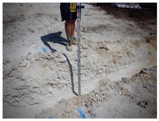
Plate 4. Prepared surface with foundation trenches marked out (looking NE)
